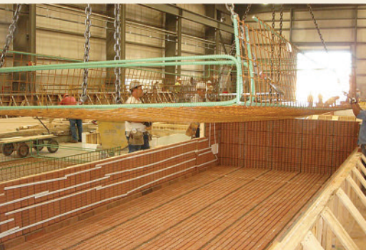
Genuine Glen-Gery clay thin brick product placed in liner and readied for initial pour.
